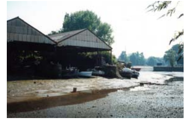
Brentford has the potential to form a major centre for small-scale water based industrial activity
