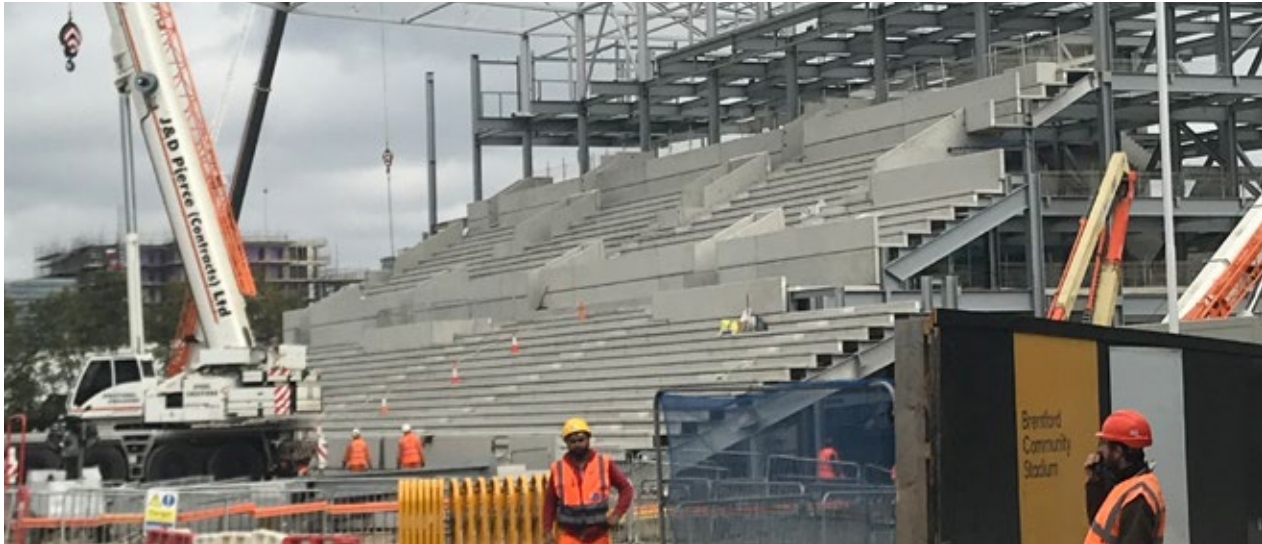
Photo of the south stand steel frame and terracing (October 2018)
